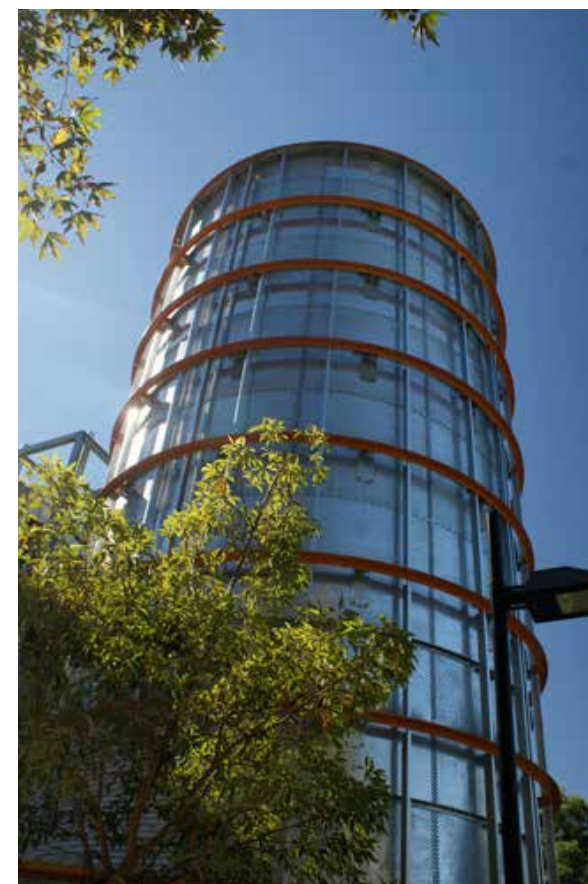
Thermal Energy Storage Tank, Macquarie University
