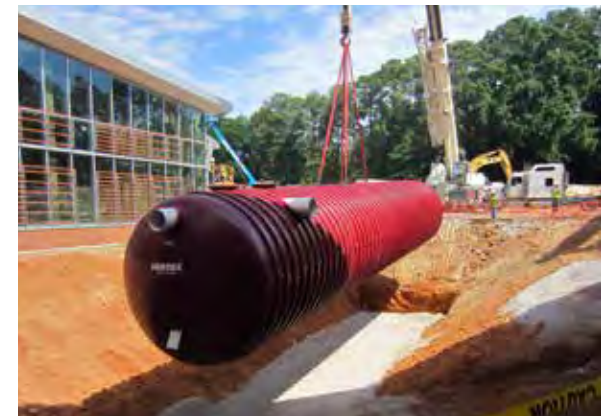
Water Cistern Installation, Talley Student Union, NC State
